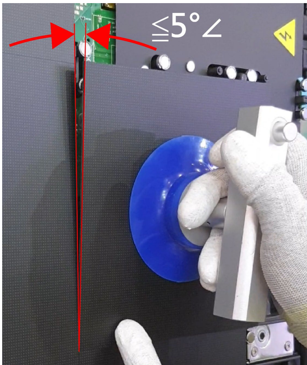
Illustration of the correct operation for installing LED panels.
